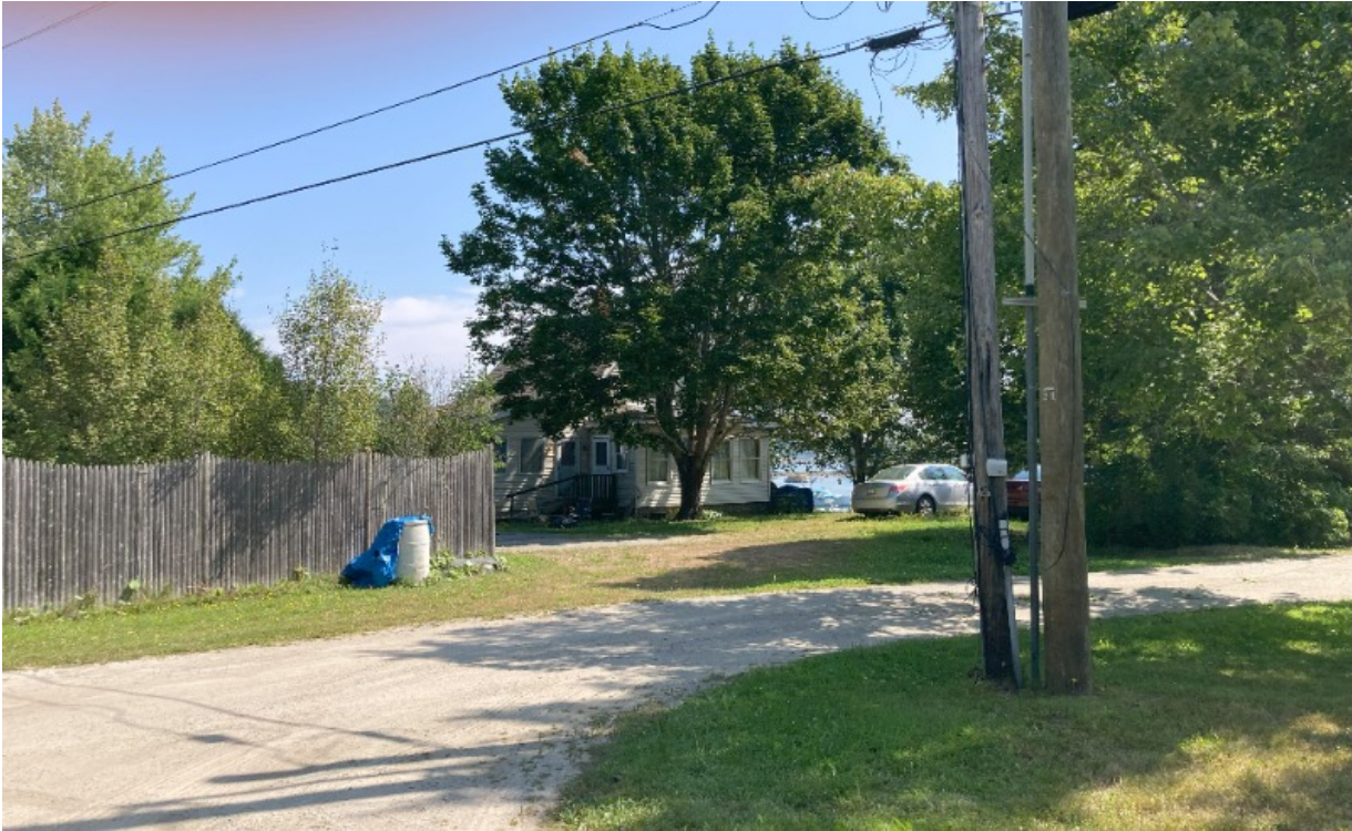
Existing residence for be removed
