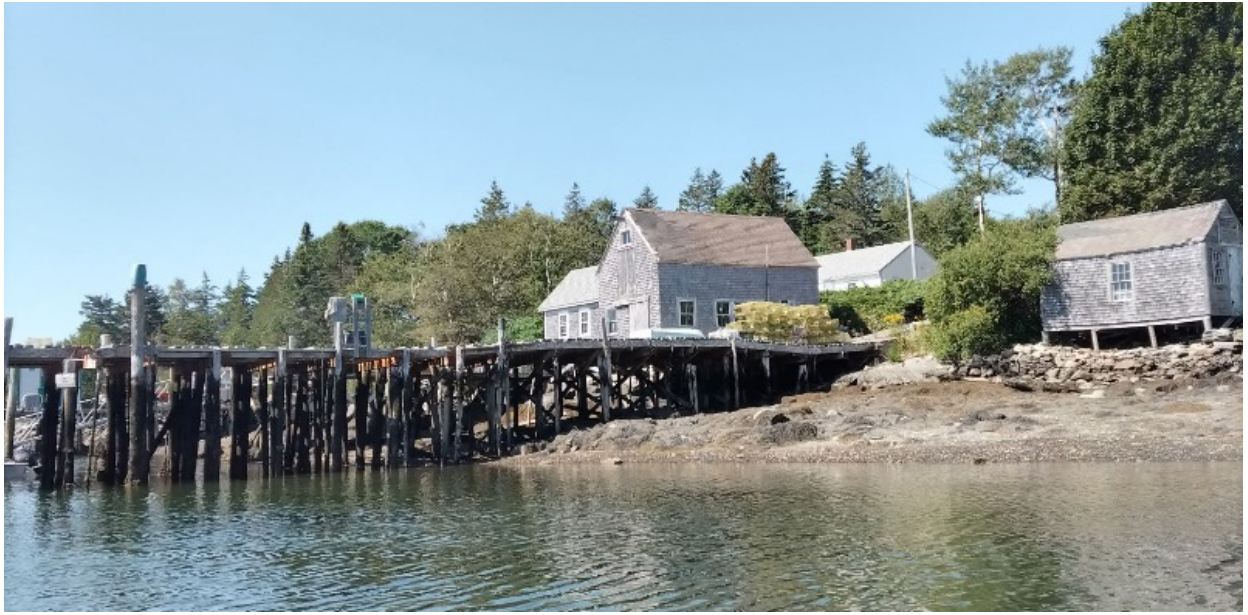
Existing wharf to be removed and replaced by launch ramp - current slope shows how this can be achieved with minimum disturbance
