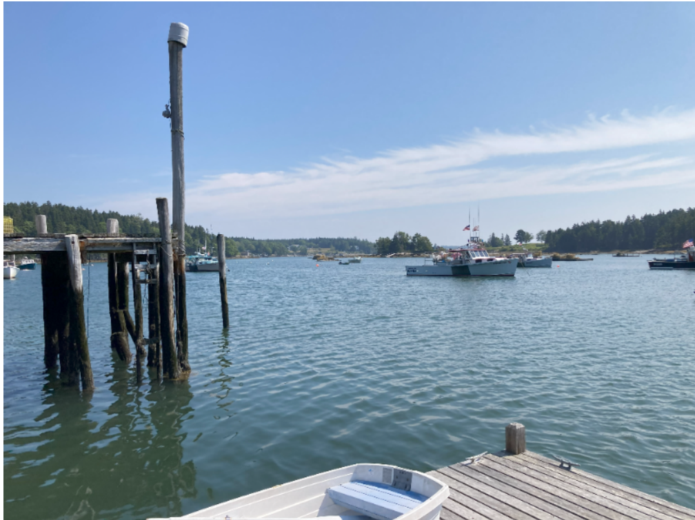
Harbor view from neighboring float showing end of existing dock
